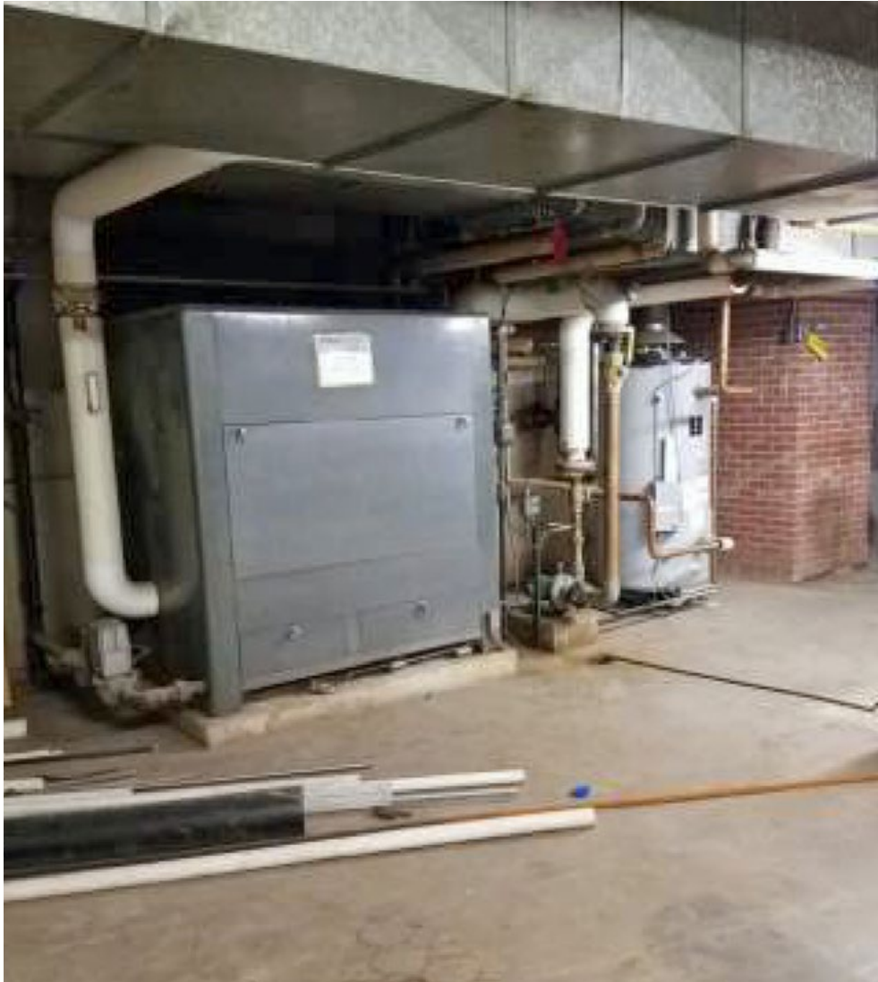
1960s Boiler, Water Heater
